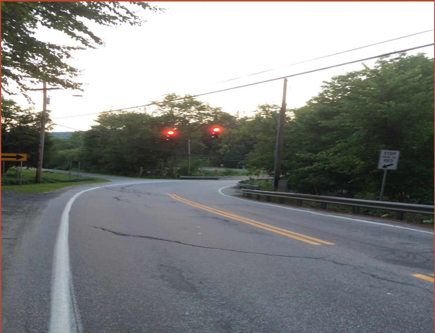
North Approach (looking south)
