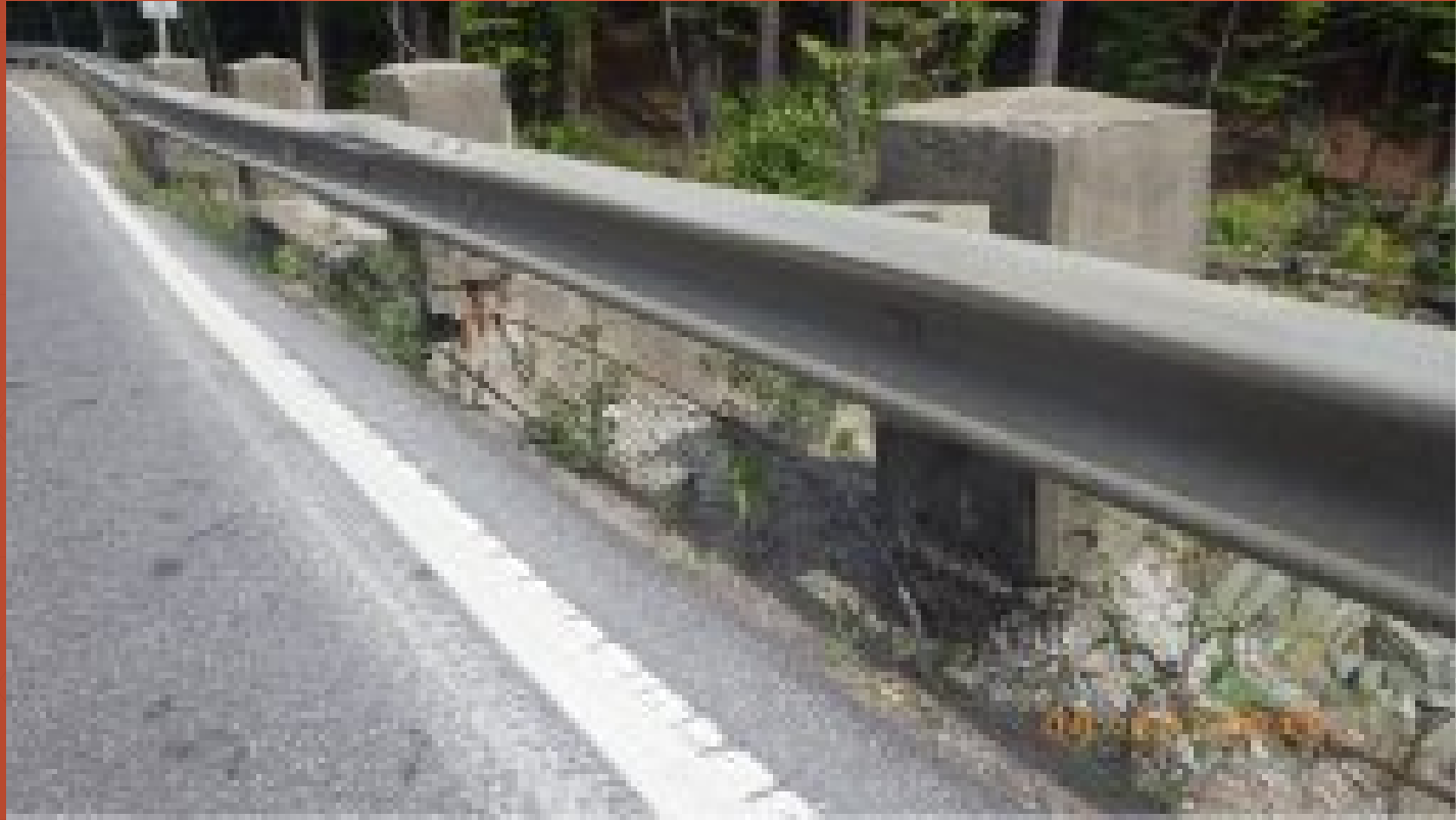
Existing Bridge Railing Posts
