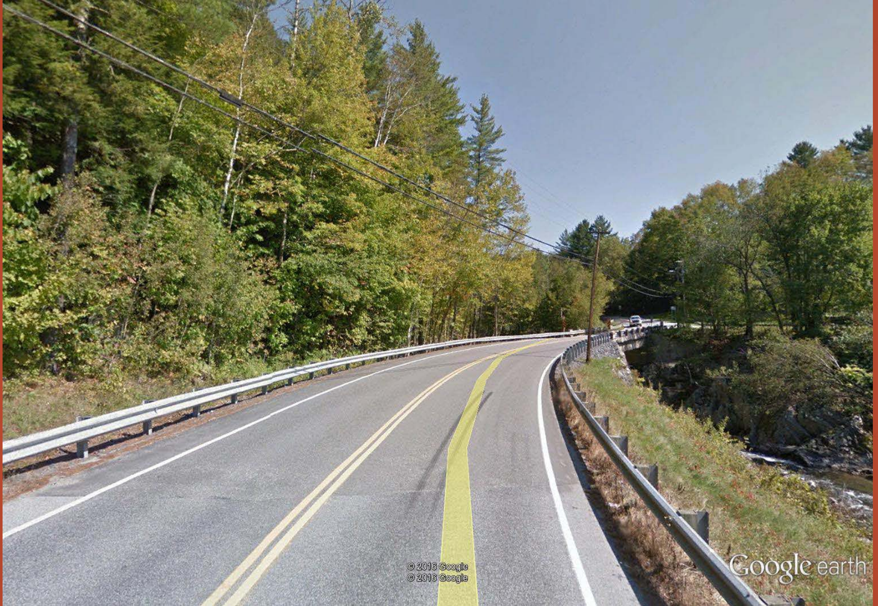
South Approach (looking north)
